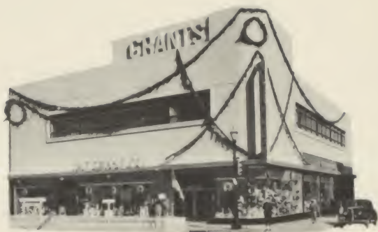
Store at Fort Worth, Texas.
